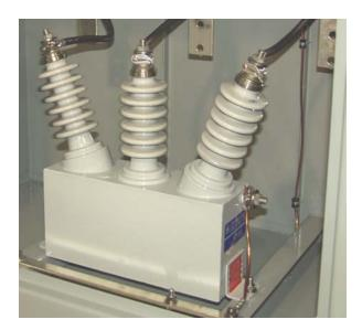
**Figure: 700-01-1** Typical 3-Phase Motor Surge Capacitor Mounted Within Motor/Generator Terminal Box
